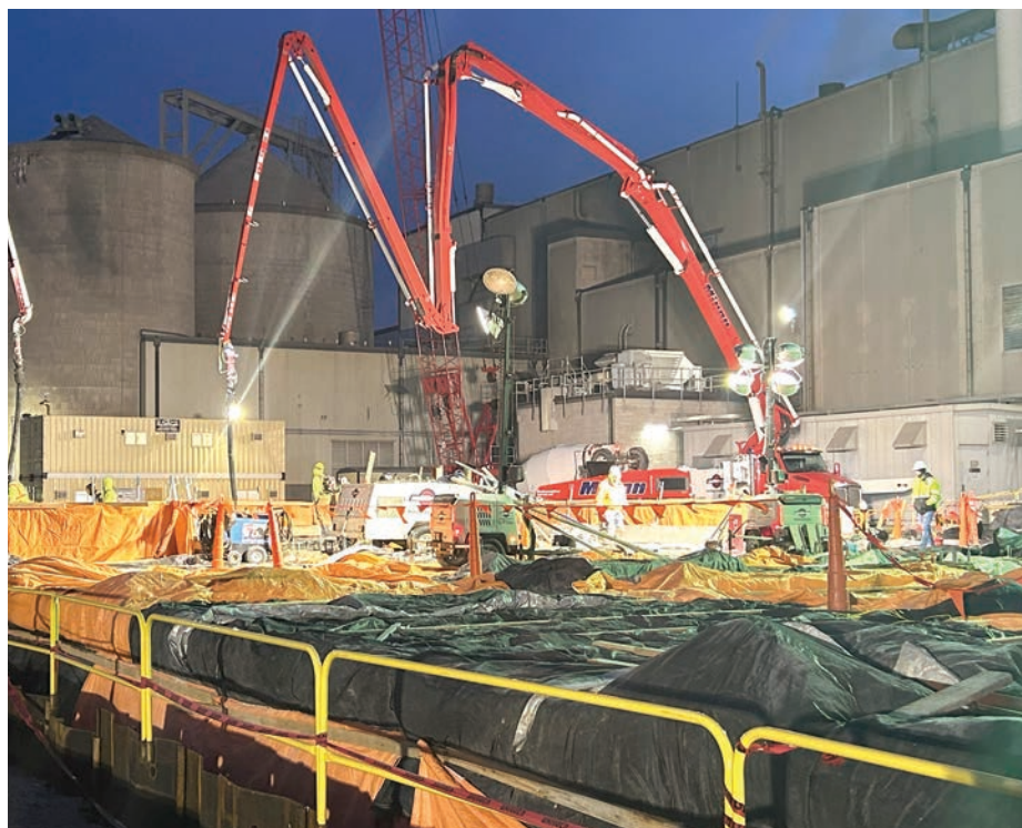
Adding to the complexity were Iowa's chilling winter temperatures, which required a special concrete thermal control plan and 24/7 monitoring.
