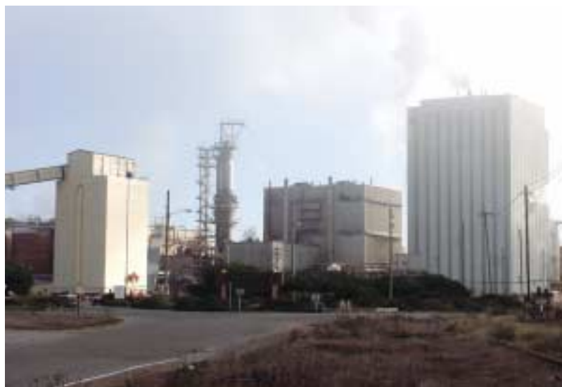
The 200,000-metric tpy mill at Samoa currently produces 10% of the world’s unbleached kraft market pulp, with a 600 (plus)-metric tpd continuous digester and a chemical recovery boiler and recovery island that was upgraded in 1990.
