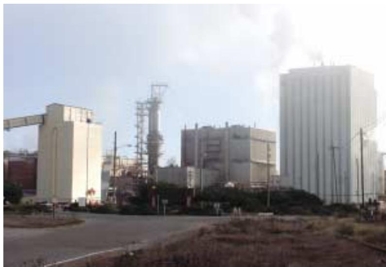
The 200,00-metric tpy mill at Samoa currently produces 10% of the world’s unbleached kraft market pulp, with a 600 (plus)-metric tpd continuous digester and a chemical recovery boiler and recovery island that was upgraded in 1990.
