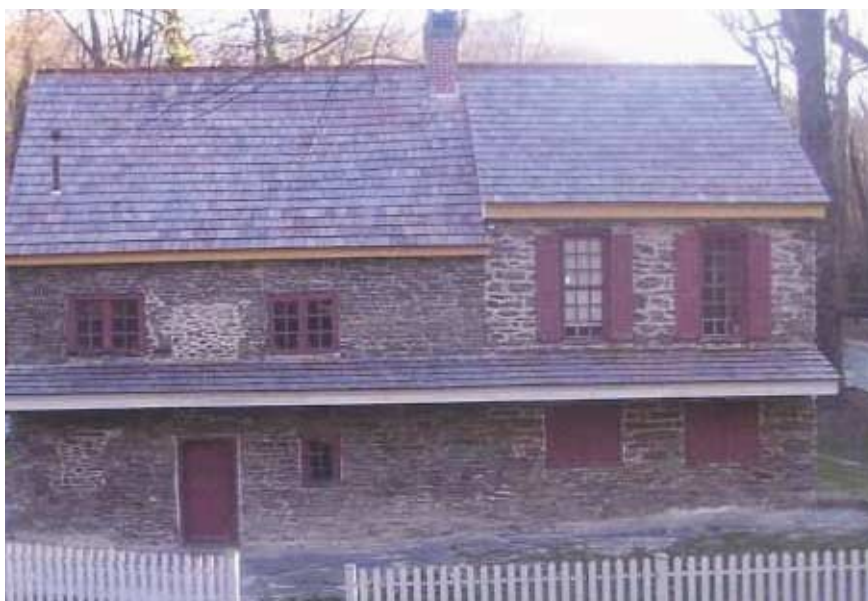
This house is from 1707. It is a National Landmark and the birthplace of David Rittenhouse (Historic Rittenhouse Town). It has an addition from 1713. The first papermill in America was at this site.
