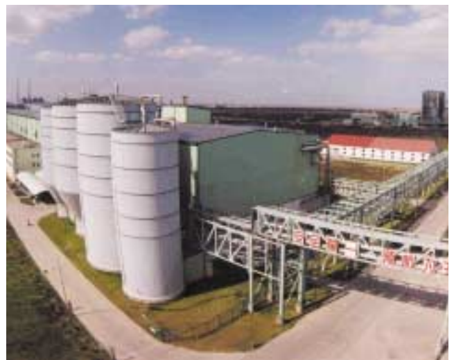
Aerial view of Changshu mill. The facility has a production capacity of 350,000 tpy of fine paper.
