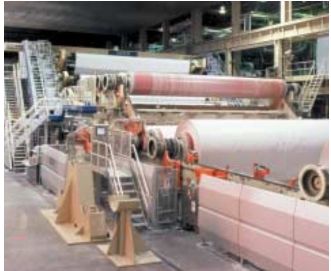
The rebuilt PM 3 has a production capacity of 330,000 tpy of No. 5 coated groundwood grades. It has a 353-in. trim and can operate at speeds up to 4,200 fpm.
